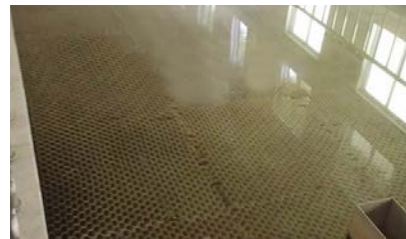
Inclined tube settler is used to purify waters in water treatment applications
